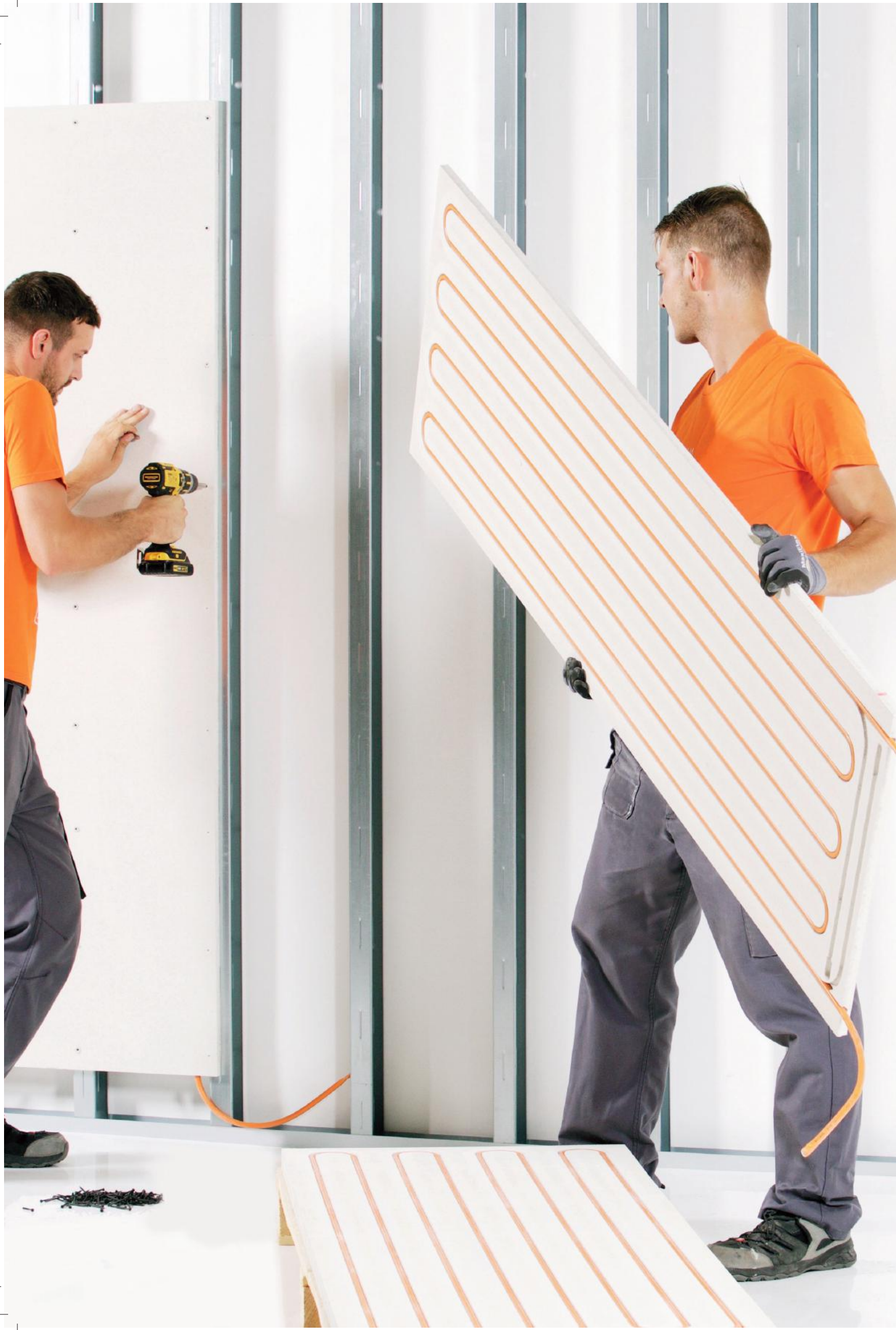
MODULAR WALL HEATING | COOLING
