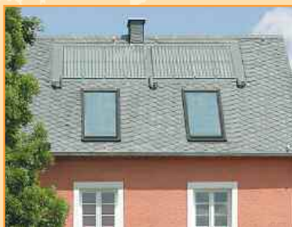
Hardly visibly in-roof mounted TUBO modules, Germany
