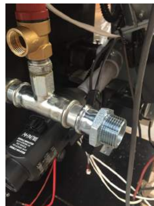
Flow connection from boiler. 1"/DN25
