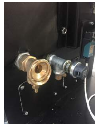
Return connection to boiler via 1"/ DN25 pump valve.
