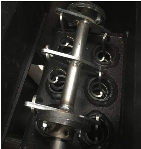
Boiler Heat Exchanger Cleaning
