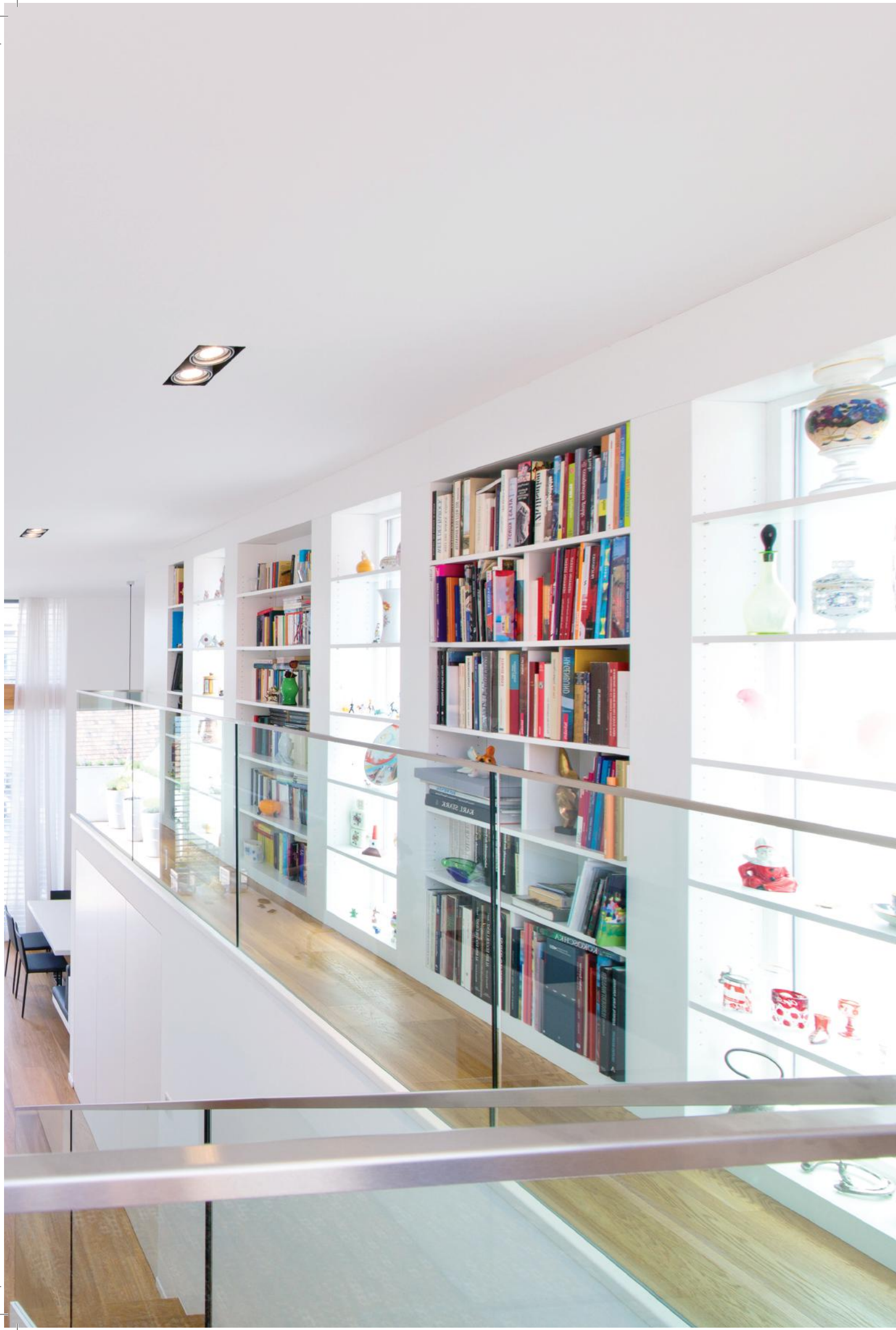
MODULAR CEILING COOLING | MODULAR CEILING HEATING
